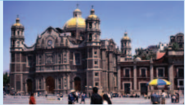
FIGURE 7-7 The sinking of the land is causing this church in Mexico City to lean.
